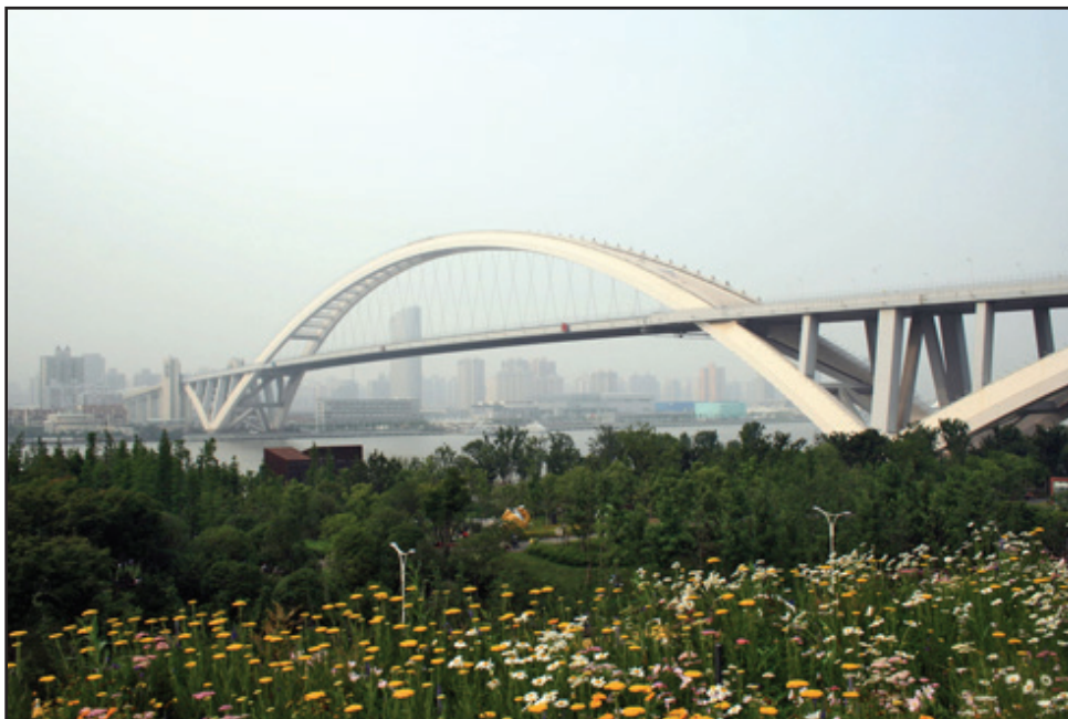
Lupu Bridge, 550-m main span, China. The Lupu Bridge is a through arch bridge over the Huangpu River in Shanghai. It connects the city's Luwan and Pudong districts. It carries six lanes of the North-South Elevated Road, which intersects with the Inner Ring Road on the Puxi side of the river. It was designed by the Shanghai Municipal Engineering Design Institute, and built by the Shanghai Foundation Engineering Co. of the Shanghai Construction Group. It was completed in 2003. It is a popular tourist attraction. Visitors ride an elevator from the bridge's base to the deck, and then climb 327 steps along the arch to an observation deck. Wikimedia Commons
