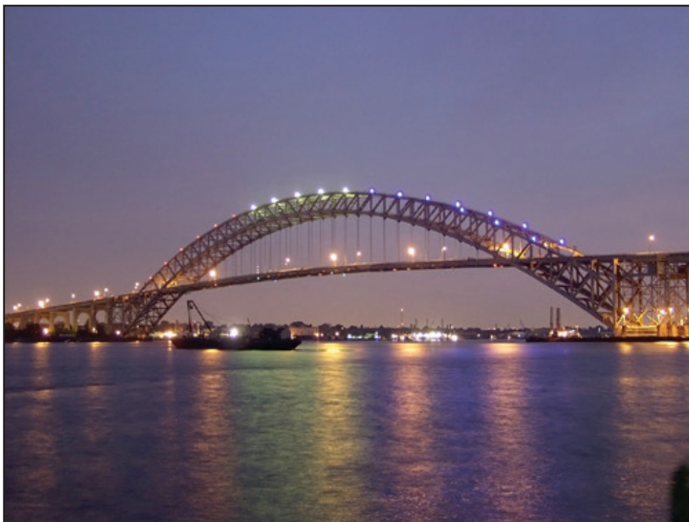
Bayonne Bridge, 510-m main span, New York-New Jersey. A steel arch bridge, the Bayonne Bridge links Bayonne, N.J., with Staten Island, N.Y. It was designed by noted bridge designer Othmar Ammann and architect Cass Gilbert, and opened in 1931. It spans the Kill Van Kull, a tidal strait connecting Newark Bay with Upper New York Bay, which is the main entryway for container ships destined for Port Newark. In order to accommodate larger post-Panamax ships that will be using the newly expanded Panama Canal, the Port of New York and New Jersey, the bridge's owner, is raising the bridge's roadway by 64 ft. A joint venture of Skanska Koch and Kiewit Infrastructure Co. were awarded a $743 million contract, and work began in 2013. A new roadway will be built above the existing road within the current arch structure, after which the existing roadway will be demolished. The project is expected to be completed in the summer of 2016. Wikimedia Commons
